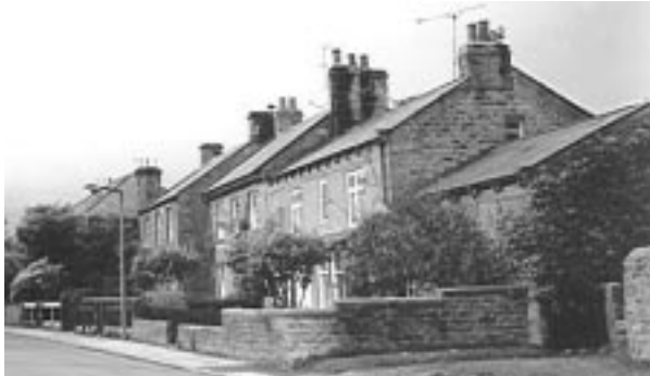
Solid chimney stacks on gable ends. Note the different pitches of these slate roofs.
