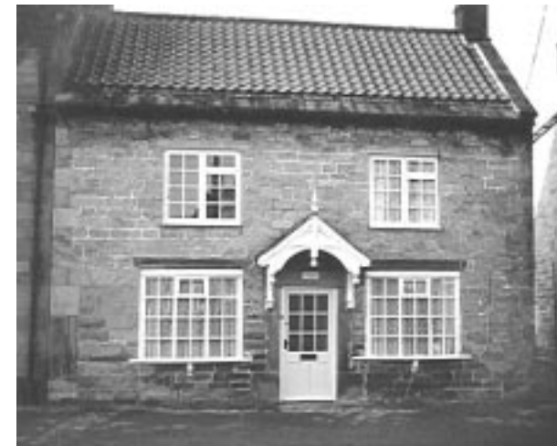
Pantile with slate edge roof. Mowbray porch. Shallow bow windows on ground floor.
