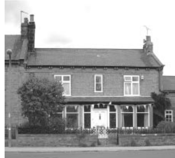
Arrowfield. The brick course below the roof shows the line of the original 'ling' roof. (Map Ref V)
