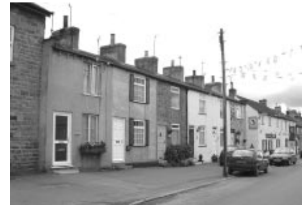
Houses in the central part of Main Street
